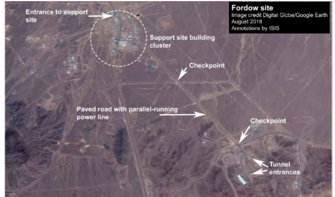
Figure 2. Overview of the Fordow facility, which includes the underground tunnel complex and the support complex.
